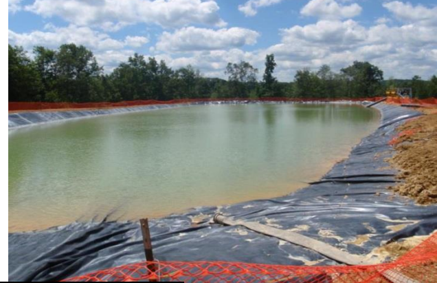
Lined Fresh Water Supply Pit, Marcellus Shale Development in PA
